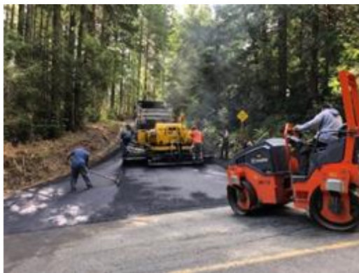
5/22/23 Begin asphalt overlay on lower Leeward from Beach
