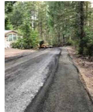
5/22/23 Crushed rock fine grading/paving prep Leeward
