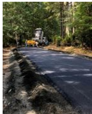
5/22/23 Paving repair/overlay on E Leeward Dr
