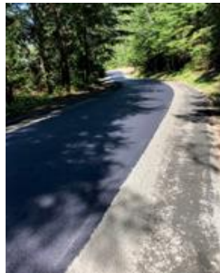
5/19/23 Paving repair/overlay on E Spinnaker Dr
