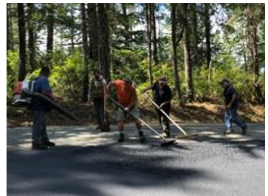
5/22/23 Handwork completing transition at upper Leeward & Beach
