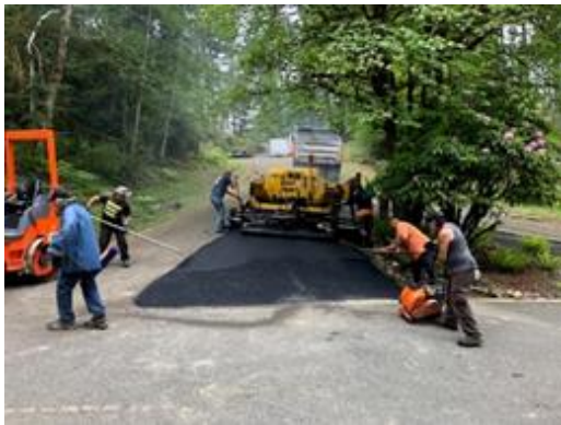
5/19/23 Paving repair around Bowsprit Island
