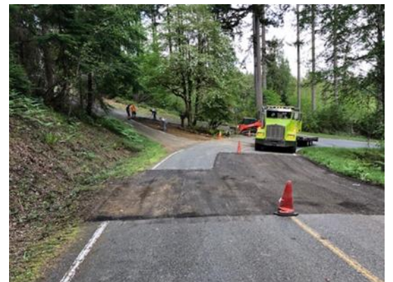
5/16 Grind out repair areas along E Beach Dr & prep for Patching
