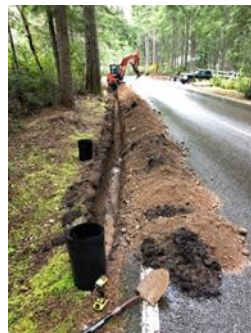
5/5 Trenching for Root Block along Beach Dr.
