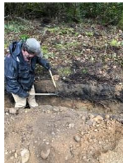
5/5 Cutting existing roots along Beach Dr.
