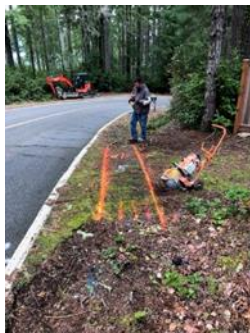
5/5 Sawcut Driveway along Beach Dr for Root Block install
