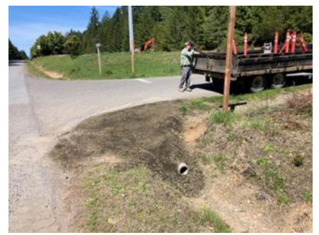
5/12 E Fairway Ln culvert extension at manzanita for enlarge street radius
