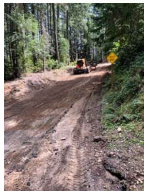
5/15 Grading along E Leeward Dr
