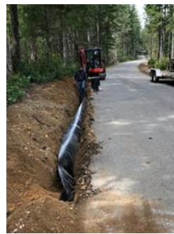
5/8 Root Barrier install along E Westwood Ln W
