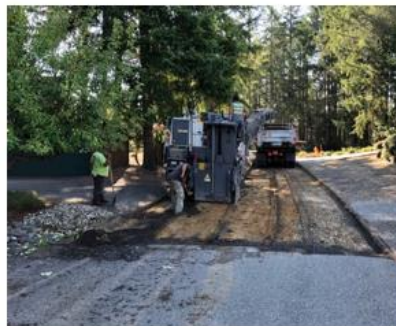
7/31/23 Grinding EWL-W Spur Road
