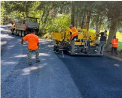
8/4/23 HMA Pre-Level on ECCDE
