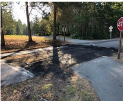
7/31/23 Grinding at DR entry
