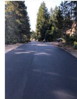
8/15/23 HMA overlay EFL
