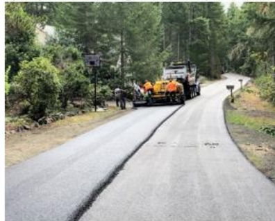
8/7/23 HMA Overlay EWL-W
