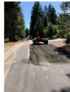
8/1/23 Crushed rock base - EFL
