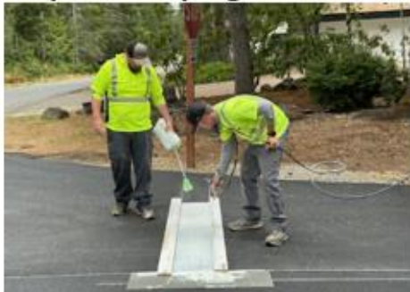
Stop Bar Striping
