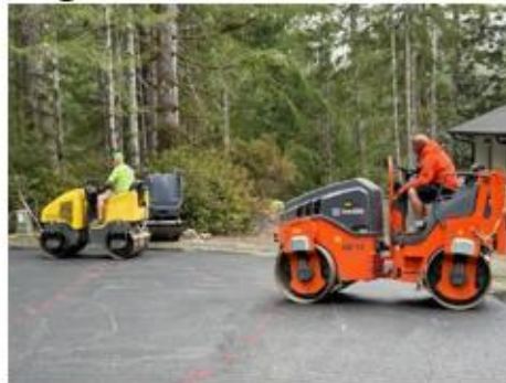
Compacting top course E Dogwood Court
