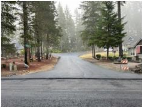
Asphalt overlay on E Vine Maple Court
