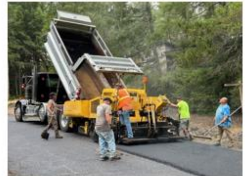
Pre-level on E Vine Maple Lane
