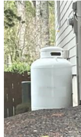
Tanks needing screening
